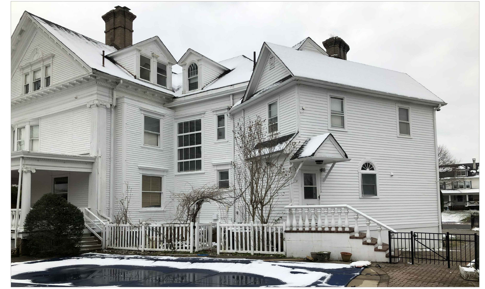
2019 VIEW OF REAR ADDITION
