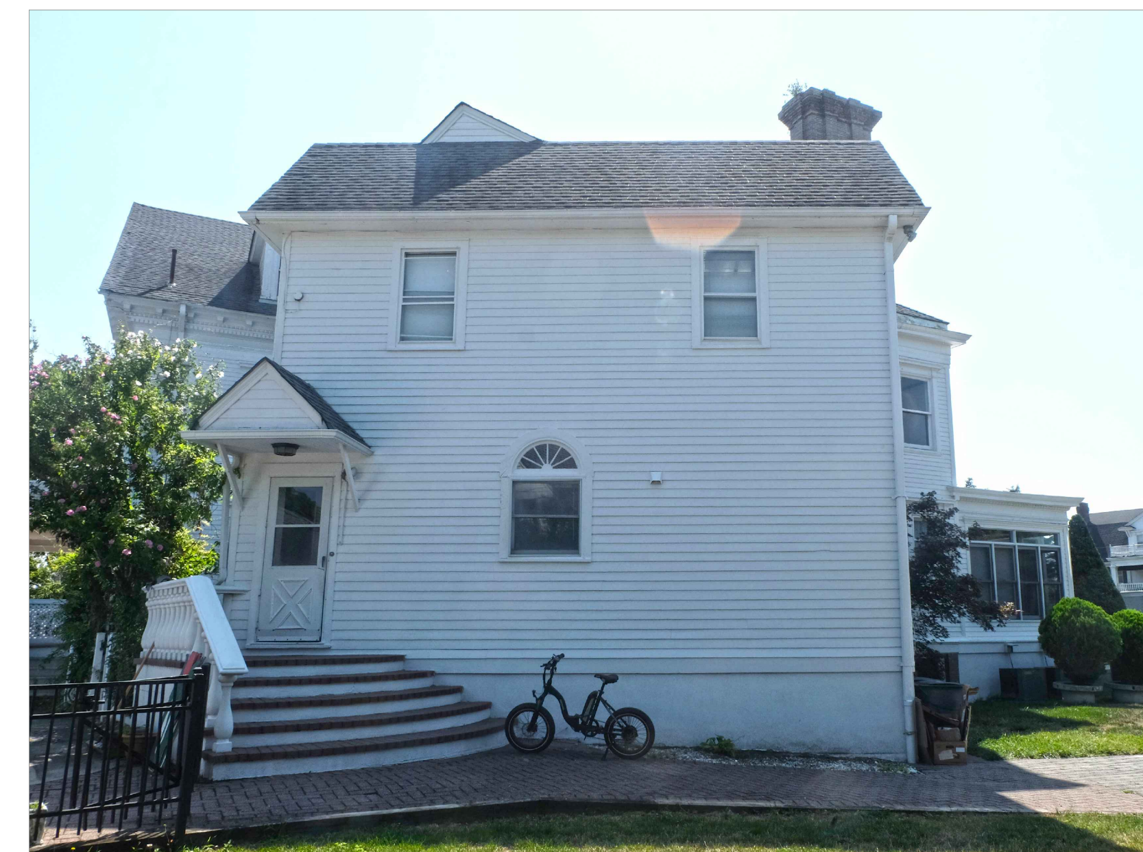
2019 VIEW OF REAR ADDITION
