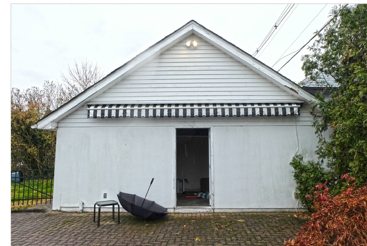
2019 CURRENT CONDITION OF EXISTING GARAGE
