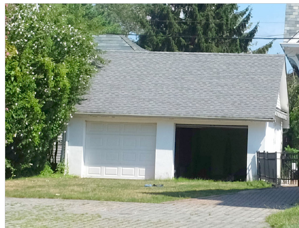
2019 CURRENT CONDITION OF EXISTING GARAGE
