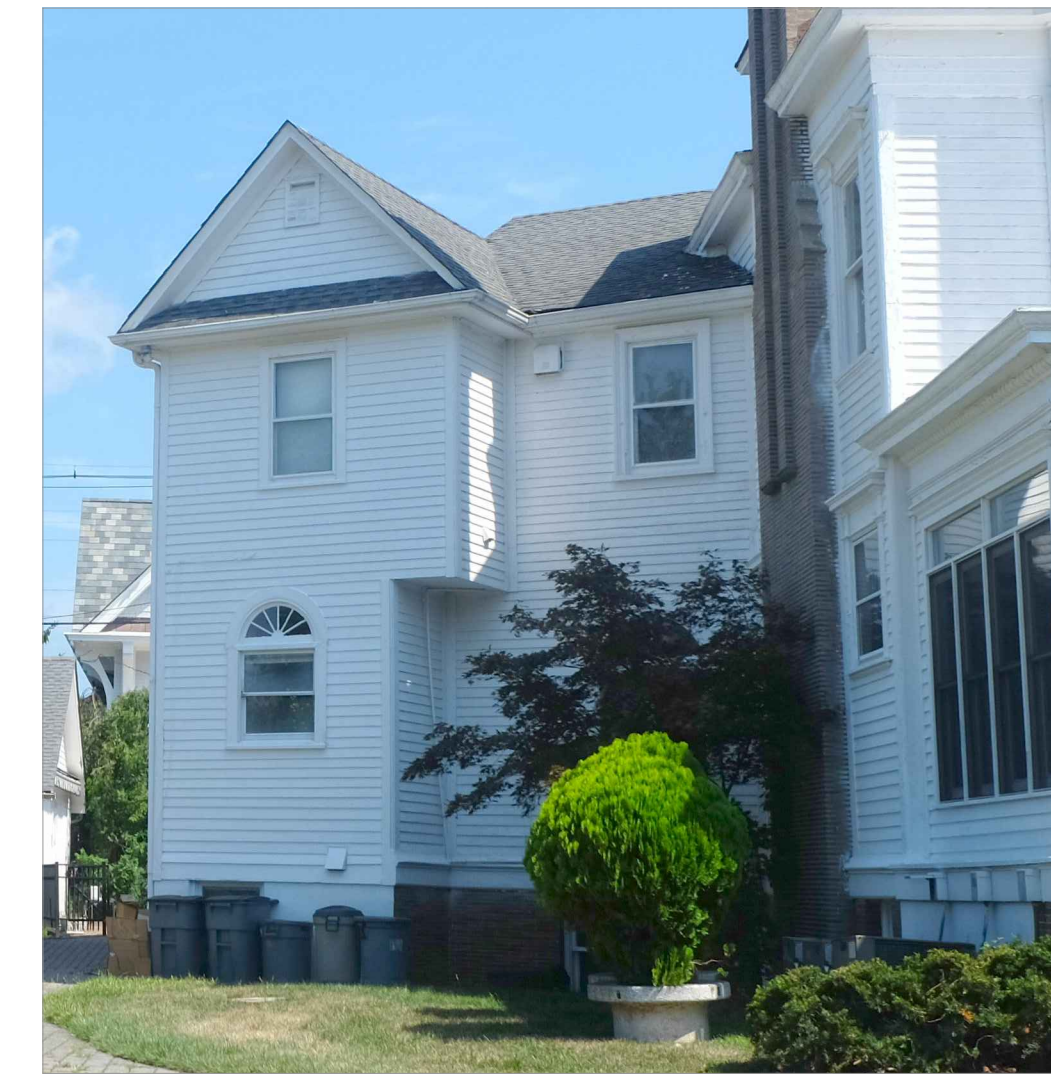
2019 CURRENT CONDITION OF HOUSE - REAR ADDITION
