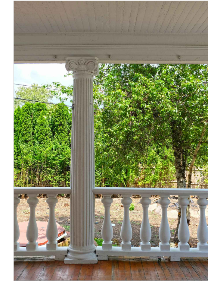
DETAIL OF CURRENT PORCH RAILING
